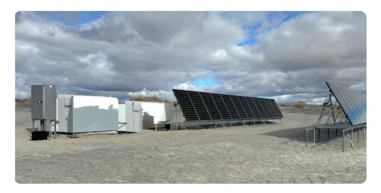
Berger Solar Electric's commitment to using top-quality products led to installing 24 Maxeon 425 W solar modules, a Sol-Ark 15K-2P-N inverter, and Discover Lithium batteries, creating a reliable and efficient energy generation and management system. The upgraded system is designed to provide several days of autonomy, ensuring uninterrupted data collection even during extended stormy weather—an essential aspect of the district's air quality monitoring mission.
